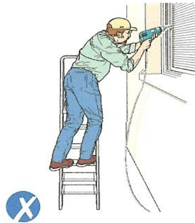
Unsafe practice: working side on to work
