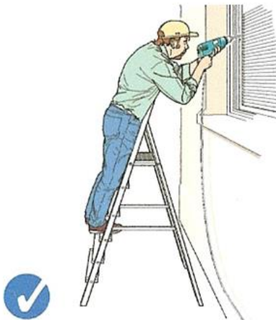
Good practice: Working face on to work & not standing above top 3 steps
